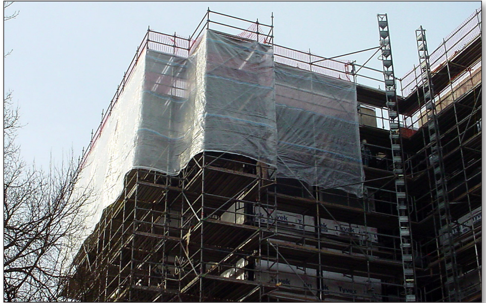
Shielding Construction During Cold Weather.
