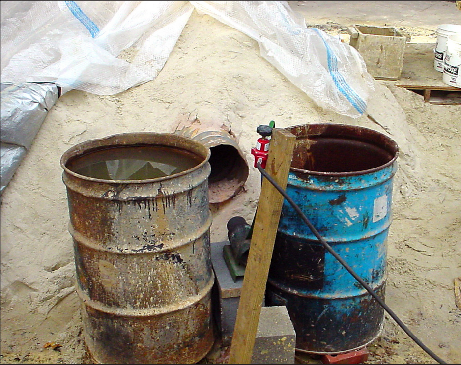
Sand And Water Heated During Construction
