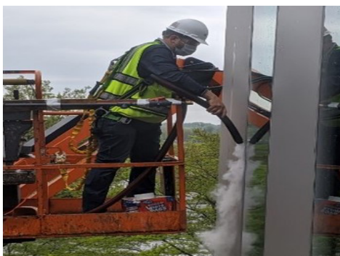
Chamber smoke tracer testing to detect potential air gaps between panels
